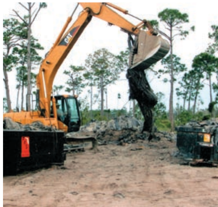
The removal of temporary roads constructed from tire mats is the last remaining heavy equipment operation.
